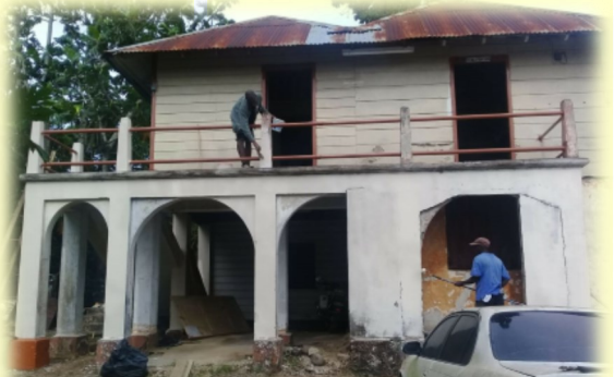
The team refurbishing the Chapelton Police Station
