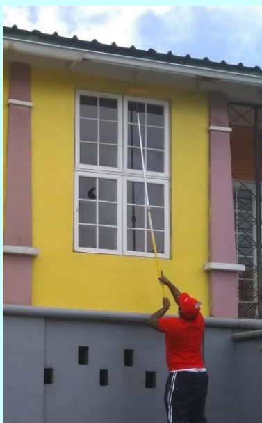
A Digicel employee paints an external wall.
