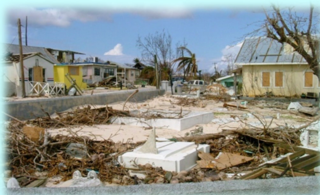
Bodden Town in Grand Cayman after Hurricane Ivan September 2004
